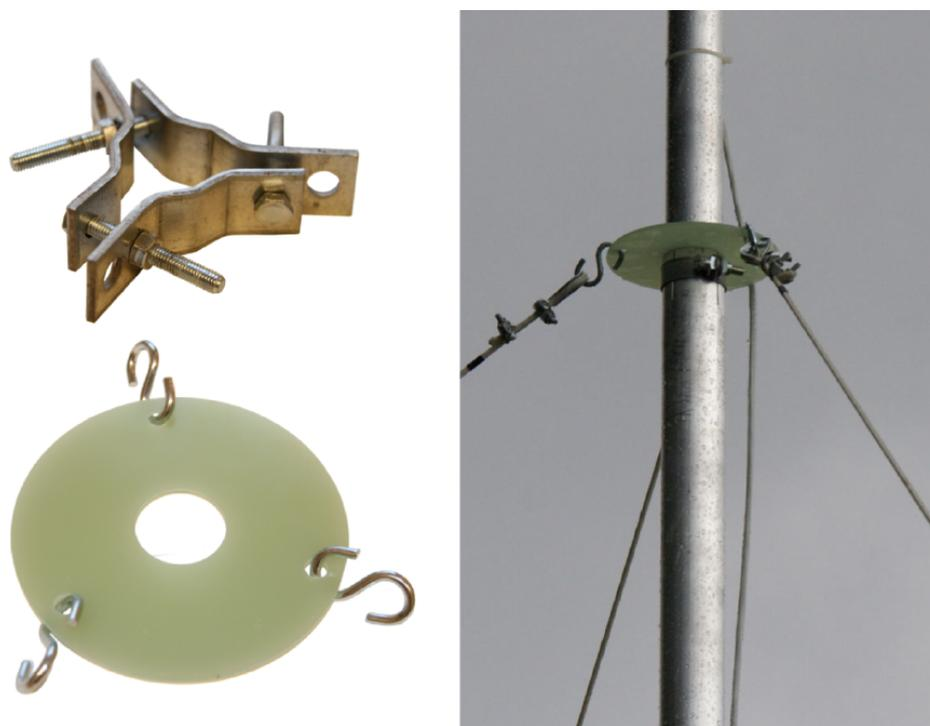
**Figure 5.12:** Primarily used fixedly mounted threepart guying clamp and its replacement part, a movable guying clamp to prevent torsion of mast.
